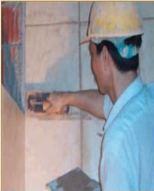
1. Spreading grout by using a soft trowel
