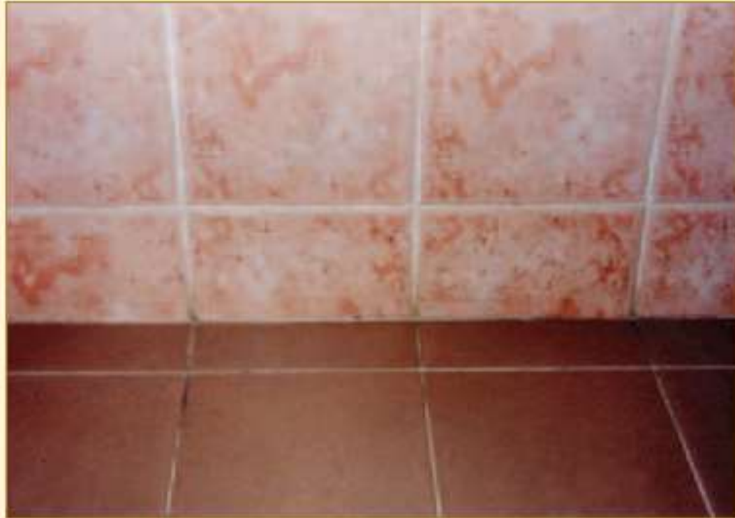
Joints aligned with wall tiles
