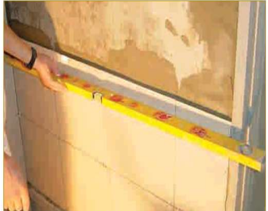
2. Checking level of tiles using spirit level
