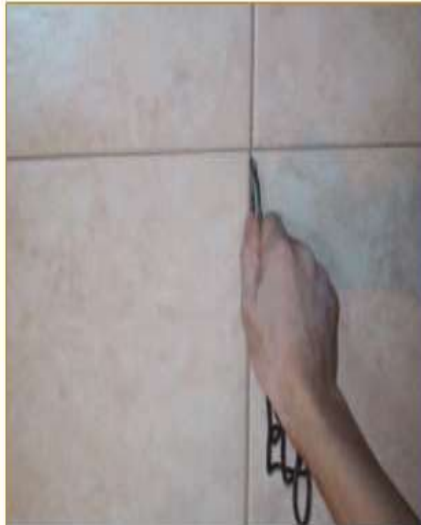
2. Removing excess grout
