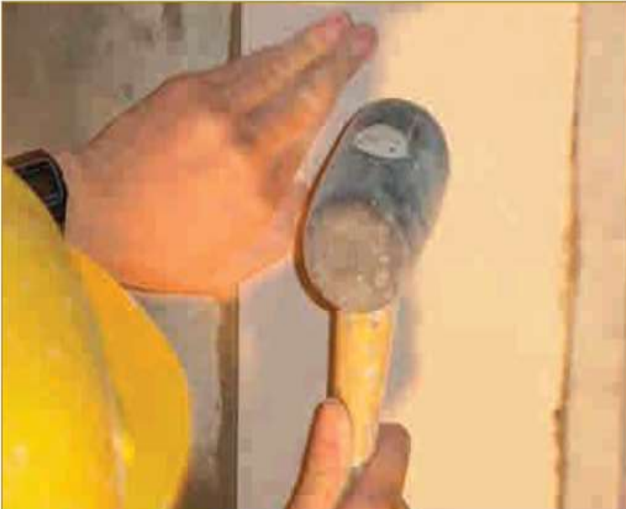
1. Tapping tile onto uniform position
