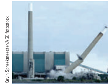
Figure 10.13 (Conceptual Example 10.5) A falling smokestack breaks at some point along its length.
