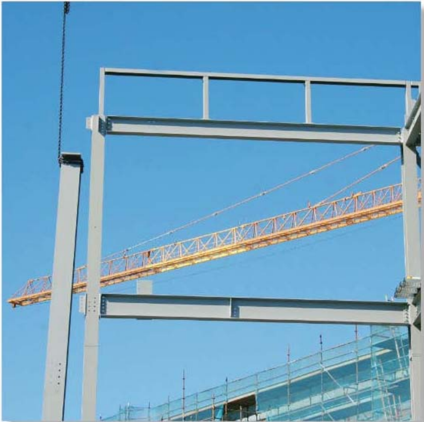
Beams are important structural members that are used to support roof and floor loadings.
