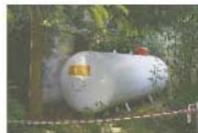
Cylindrical pressure vessels, such as this gas tank, have semi-spherical end caps rather than flat ones in order to reduce the stress in the tank.
