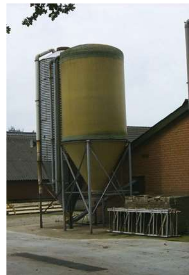
The volume of fertilizer contained within this silo can be determined using the second theorem of Pappus and Guldinus.
