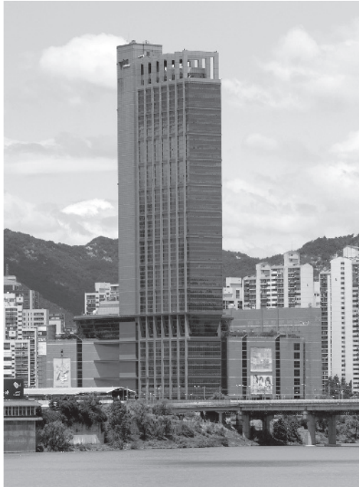
FIGURE 6.3 Vigorous exercising on the 12th floor likely led to mechanical resonance of the building triggering a two-day evacuation. (Photo courtesy of Truth Leem/Reuters.)
