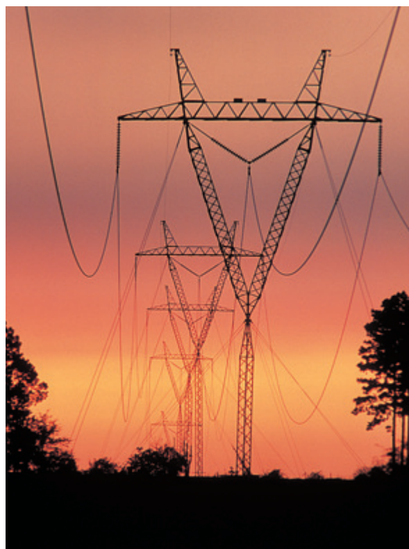
Figure 16 Power companies transfer electrical energy at high potential differences in order to minimize the I^2R loss.
