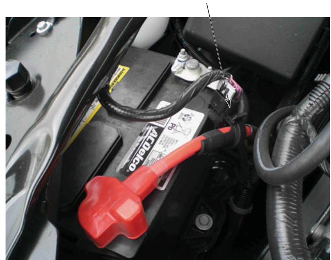
FIGURE 54-21 A Hall-effect current sensor attached to the positive battery cable is used as part of the EPM system.
