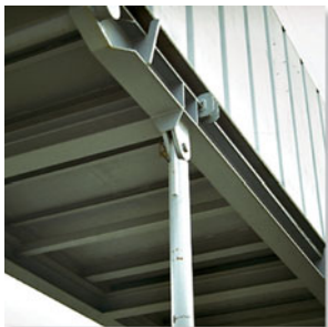
The cable exerts a force on the bracket in the direction of the cable. (1)
