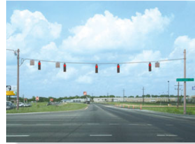
Each of the cable segments remains approximately straight as they support the weight of these traffic lights.
