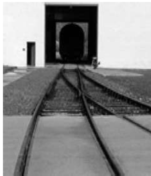
(a) Railroad tracks
