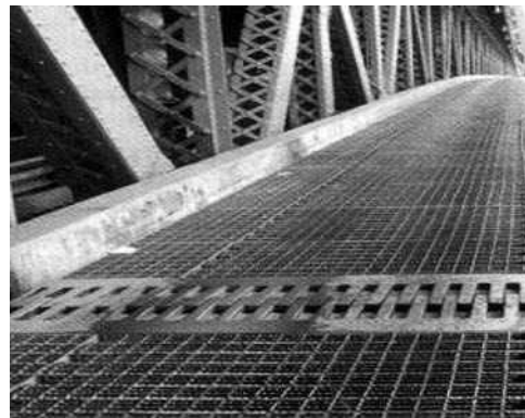
(b) Bridge expansion joint
