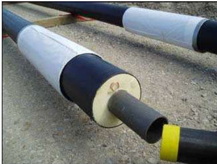
Pipes for district heating with hot water.
