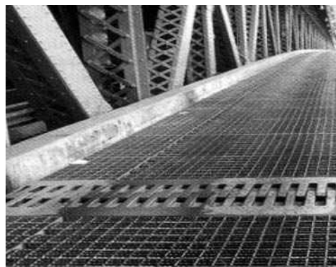
(b) Bridge expansion joint
