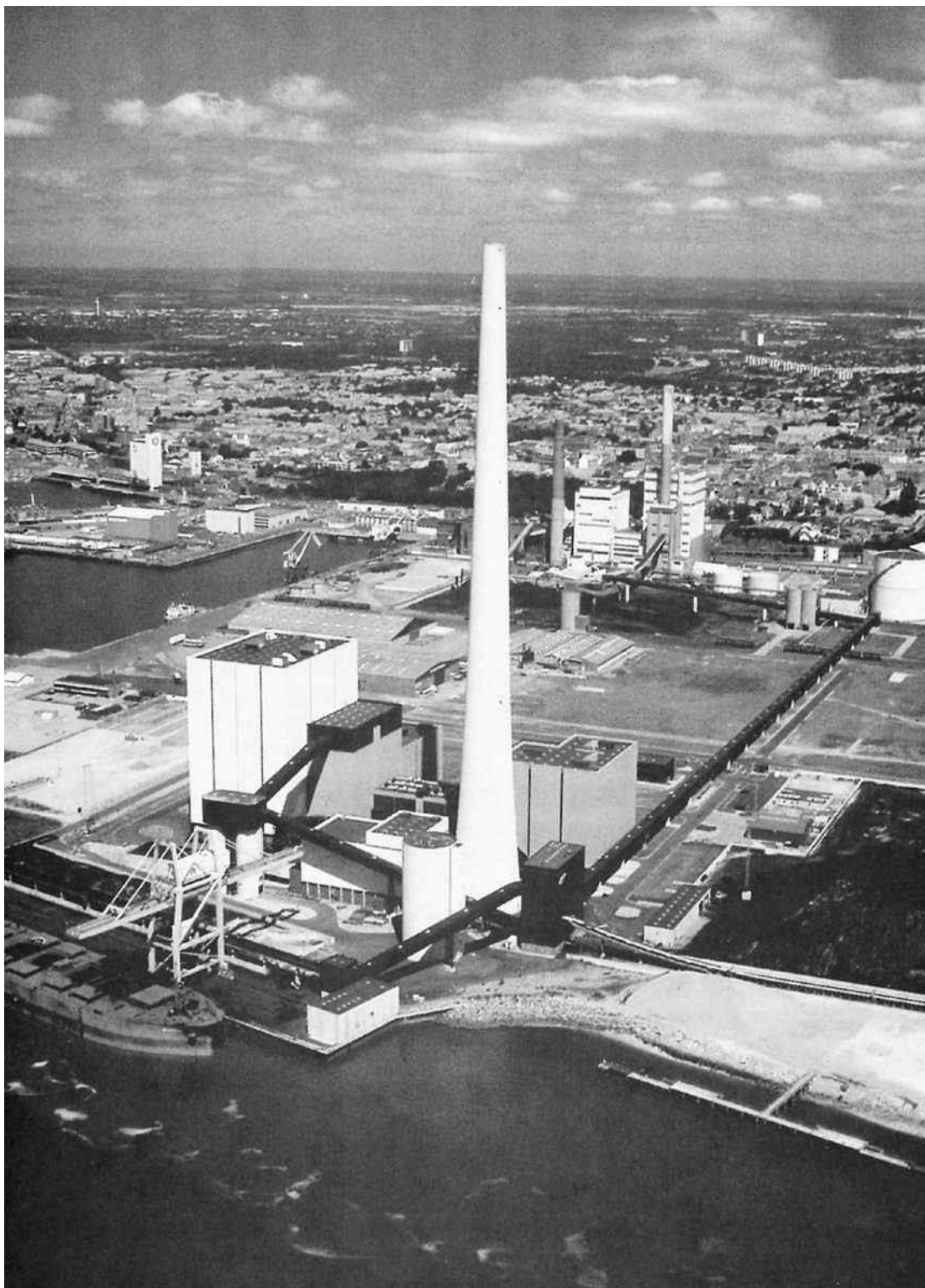
FIGURE 1.2 The Esbjerg, Denmark, power station. (Courtesy Vestkraft 1996.)
